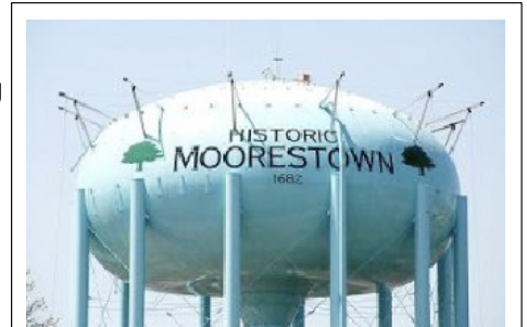
Church Street water tower being painted.
